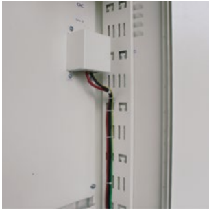
Cable Management Tray with MCB Holders
